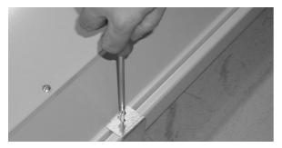
The fixing angles for the foot cover have to be screwed together with the foot elements at the back, right and left side of the bench. In this connection the bended side with the borr tape has to lie away from the assembly.
