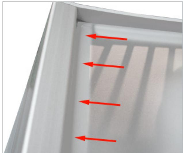
Bend the pane and push it over the right-hand edge of the aluminium section. Due to the pane being bent, it rests in its position.
